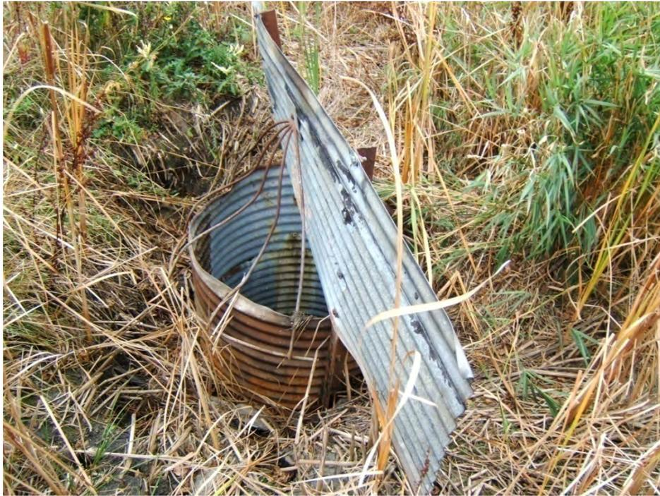
**Figure 20. Drop Structure at the Upstream End of Yaggie 1 Culvert**
